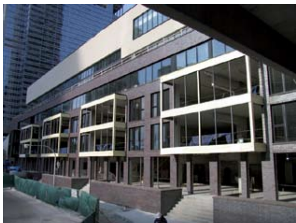
GENTILEZA STUDIO GANG ARCHITECTS
